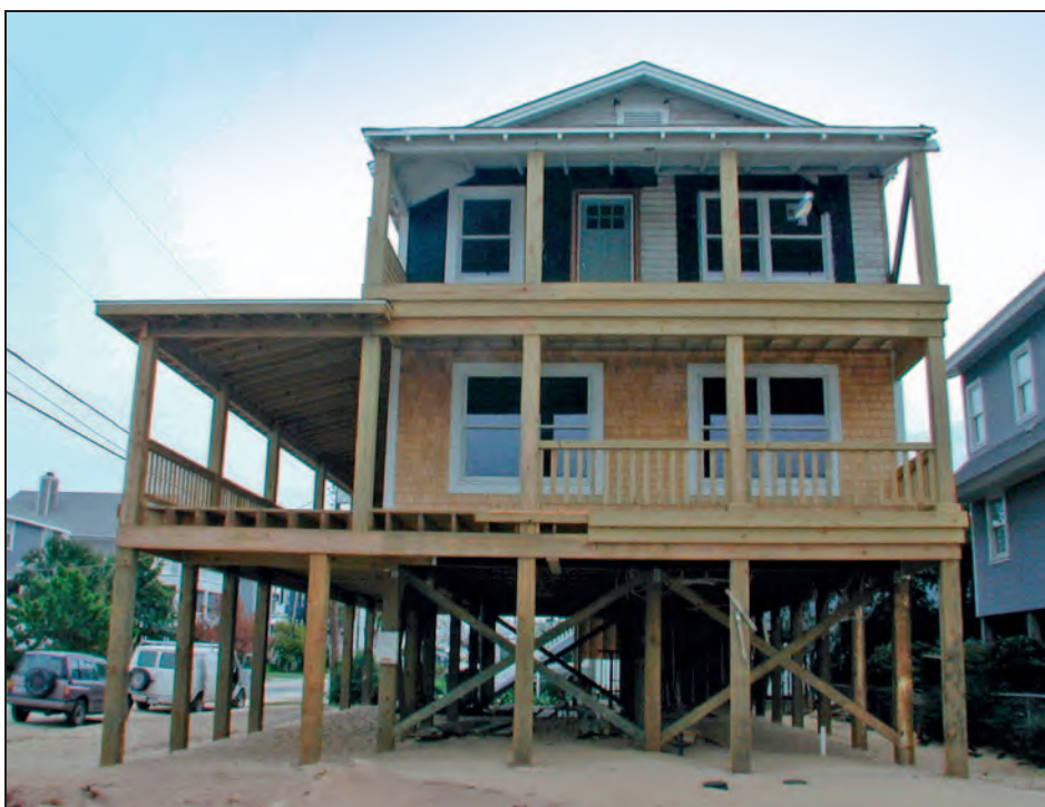
Figure 15-9. Home elevated on piles
