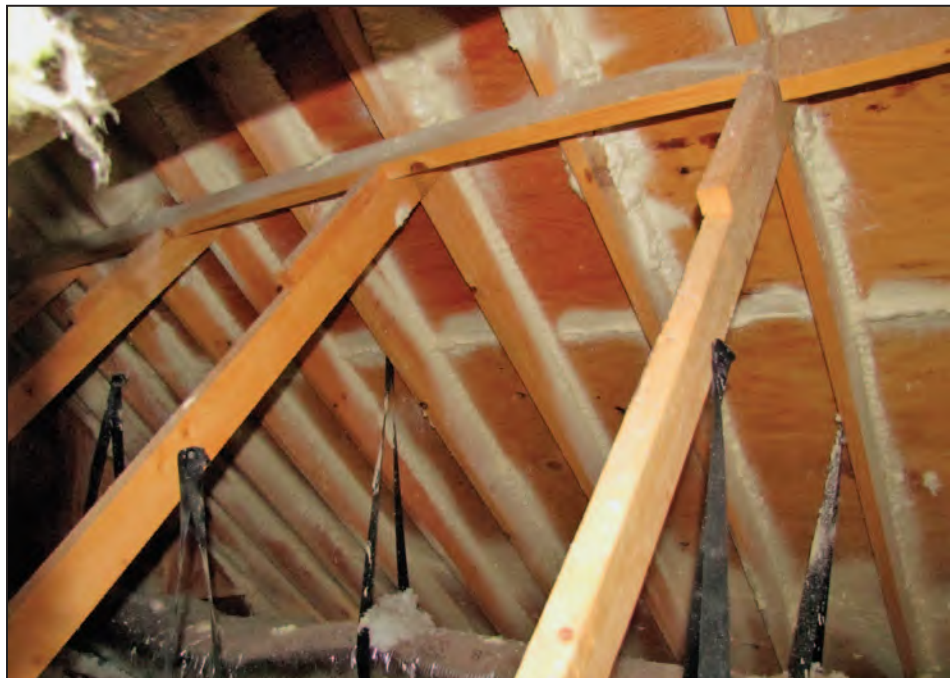
Figure 15-17. Sprayed polyurethane foam adhesive to secure roof deck panels
